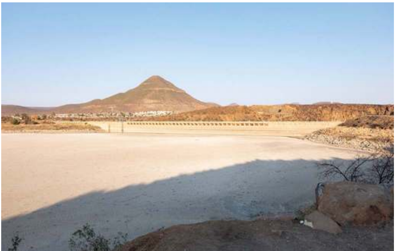
An empty Nqweba Dam, outside Graaff-Reinet. The Southern African region is projected to become drastically warmer and at the same time generally drier.
