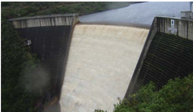
Wolwedans dam spilling
