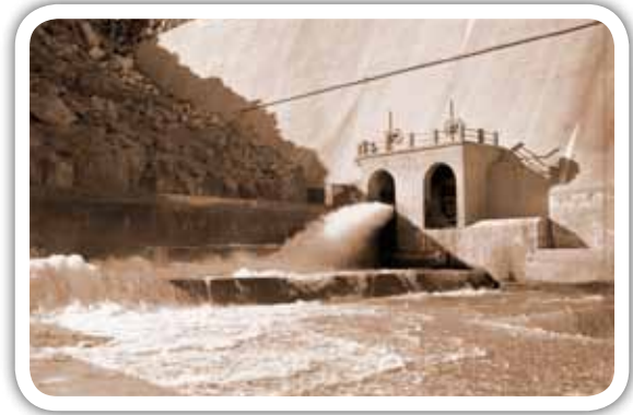
Top: The Clanwilliam Dam shortly after its completion. The original dam was a mass concrete gravity structure with a centrally situated overspill section.
