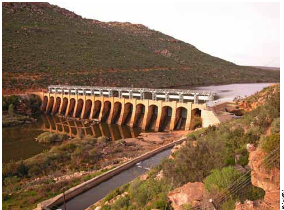
The Bulshoek Dam features 15 hand-operated gates of the Ashford type. These gates, which sit on top of the solid weir, slide in cast-iron grooves of special construction with a patented system of anti-friction rollers. Each gate is 4,6 m high and 6 m wide.
