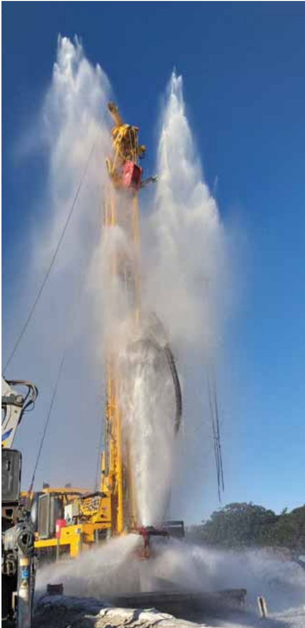
Groundwater spurts up from a depth of 265 m in the first strike at a production borehole at the Coega Kop wellfield.
