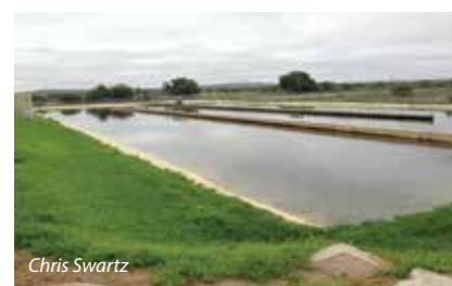
Treated effluent from Beaufort West's wastewater treatment works passes through maturation ponds before entering the reclamation plant.
