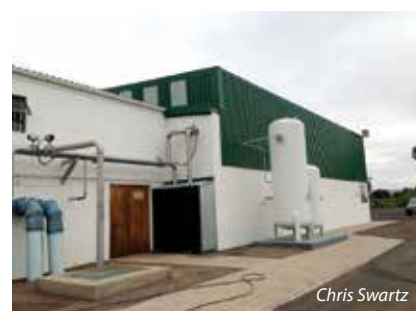
The Beaufort West reclamation plant.
